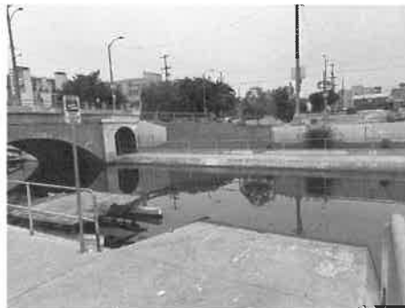
VENICE CANAL BOAT LAUNCH RAMP
