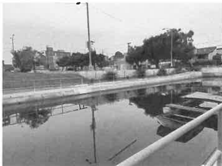
VENICE CANAL EAST WALKWAY LOOKING FROM WEST WALKWAY TOWARD S. VENICE BLVD
