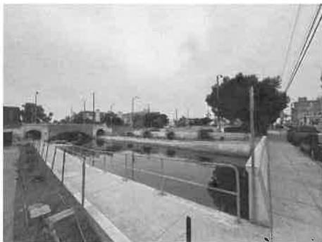
VENICE CANAL WALKWAY LOOKING TOWARD S. VENICE BLVD
